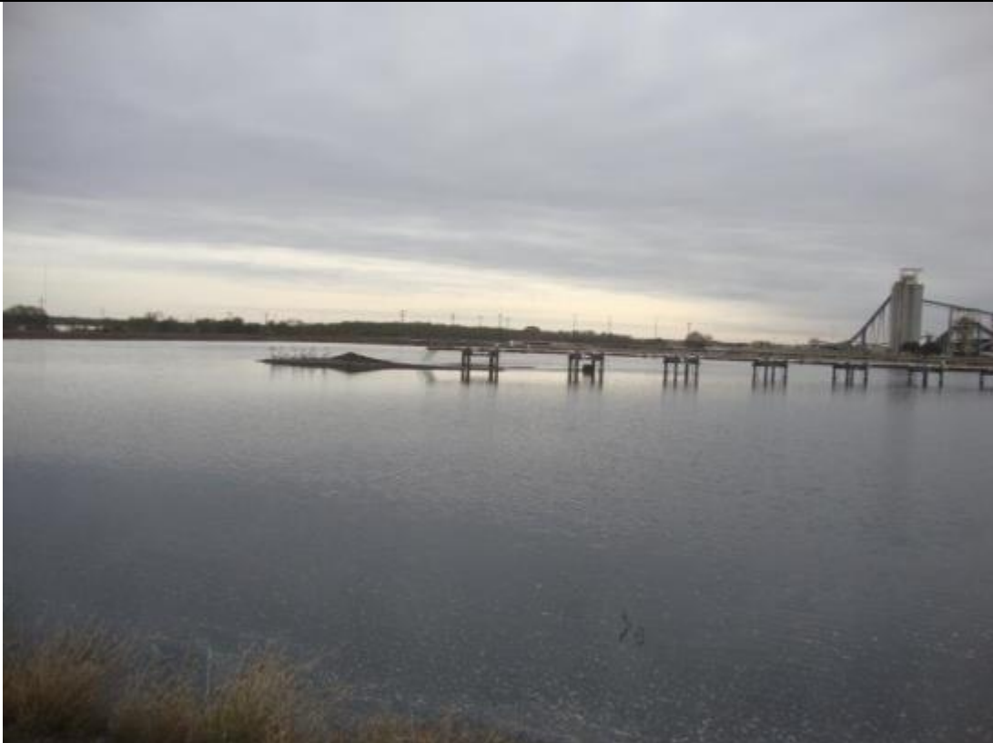
Photograph: 15 North Bottom Ash Pond – standing on northern berm – facing south. Photo taken 12/20/16.
