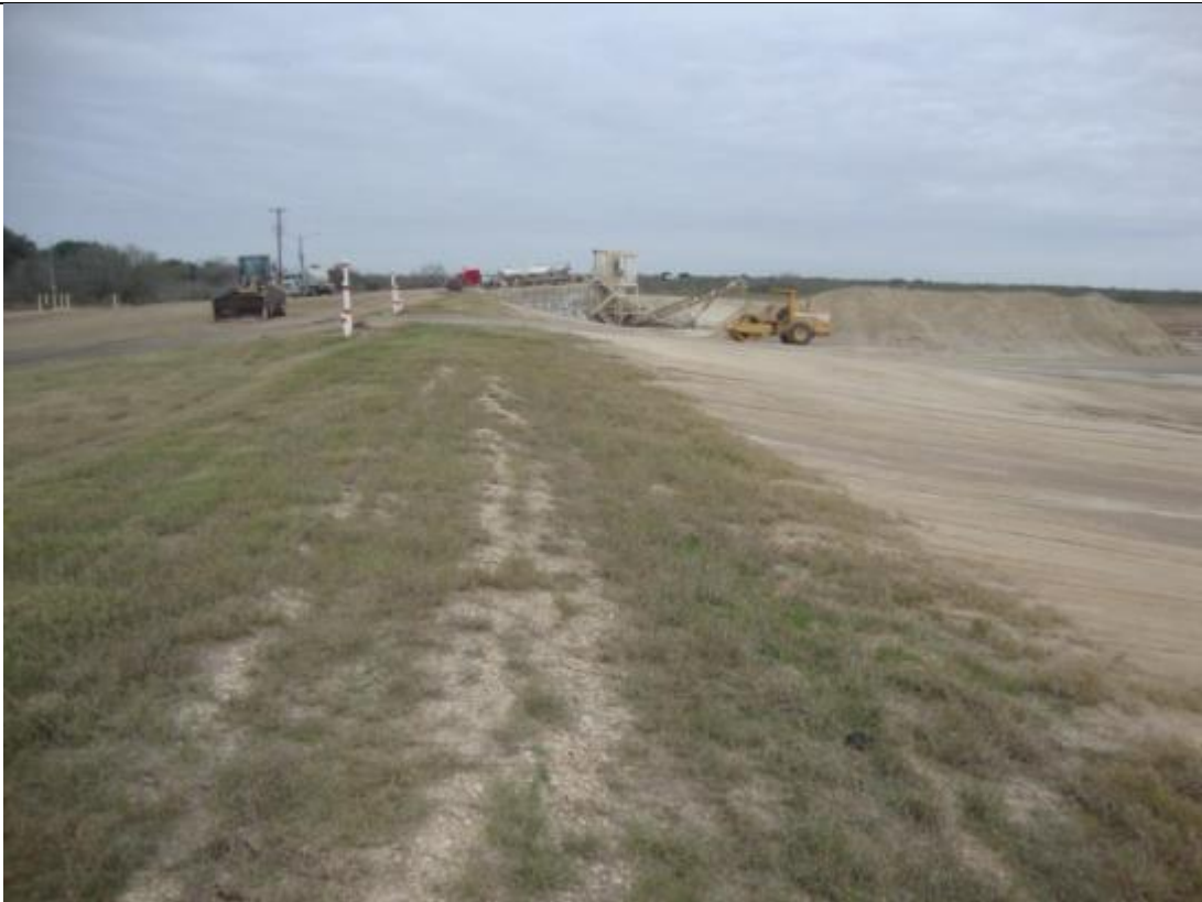
Photograph: 1 Fly Ash Landfill – standing on western berm – facing north. Mobile ash conditioning machine located in northwest corner of landfill. Photo taken 12/20/16.
