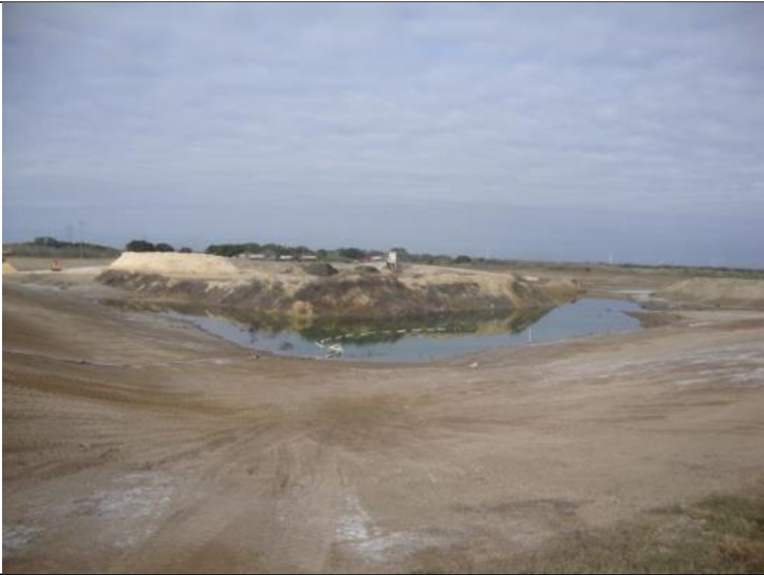
Photograph: 5 Fly Ash Landfill – standing on southeast corner of landfill – facing northwest. Rain water accumulates in southeast corner of landfill. Photo taken 12/20/16.
