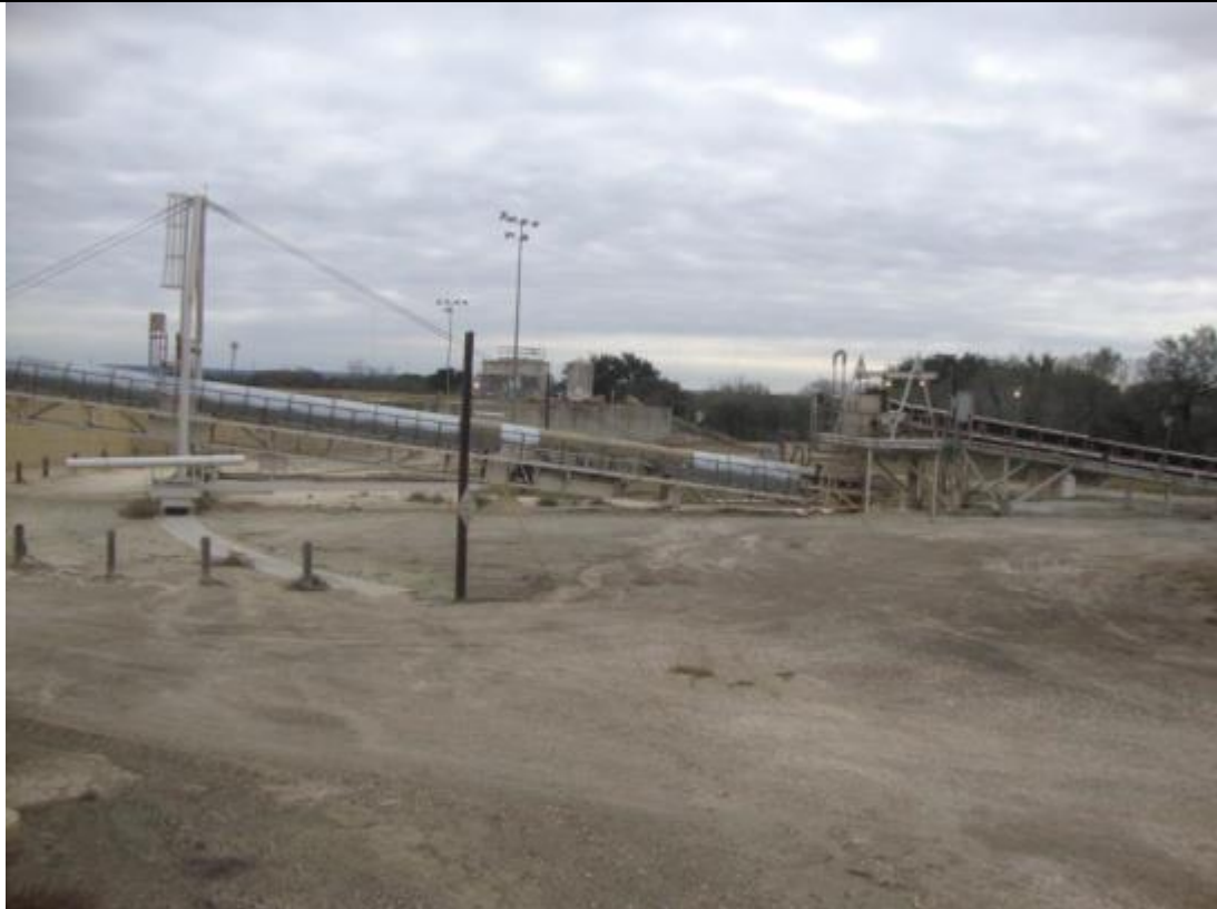
Photograph: 3 Fly Ash Landfill – standing on western berm – facing southeast. Radial stacker located in southwest corner of landfill. Photo taken 12/20/16.
