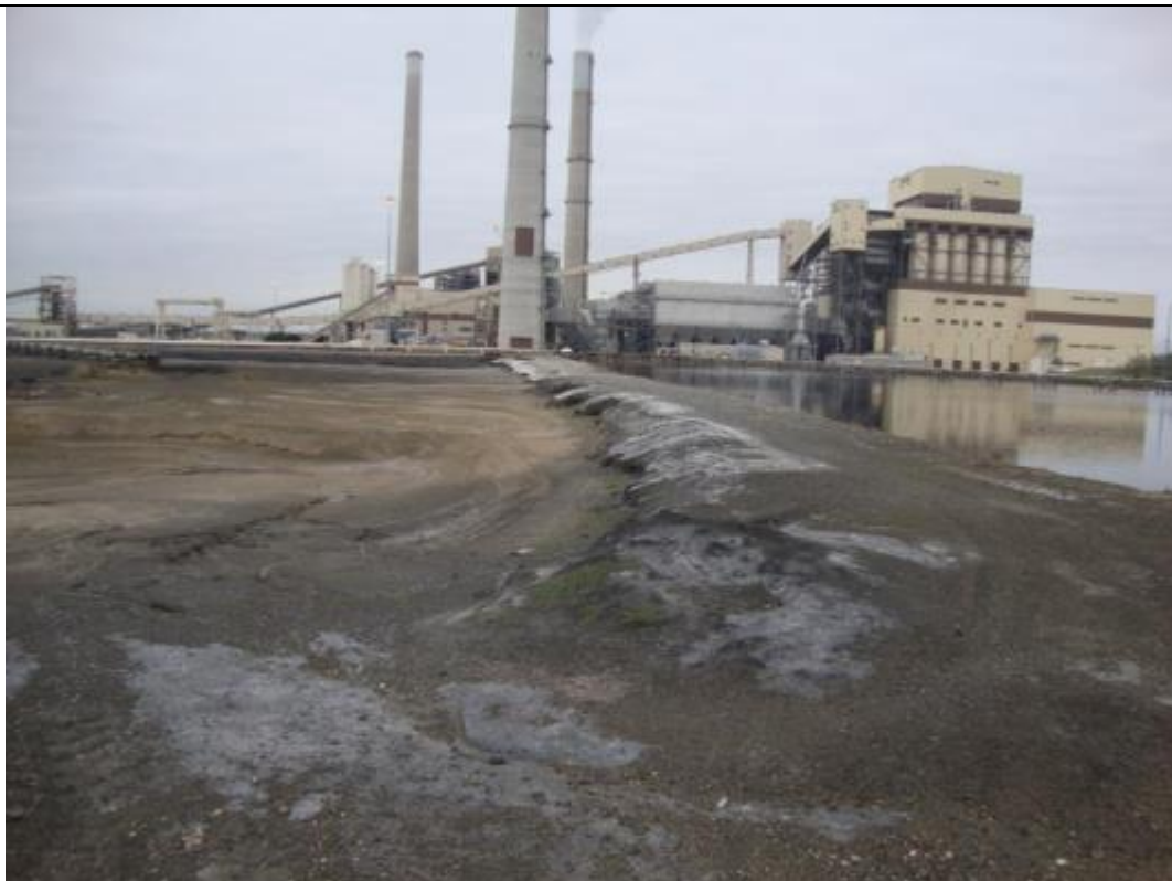
Photograph: 30 South Bottom Ash Pond – standing on northwest corner of pond – facing west. Pond was drained to remove residuals. Photo taken 12/20/16.
