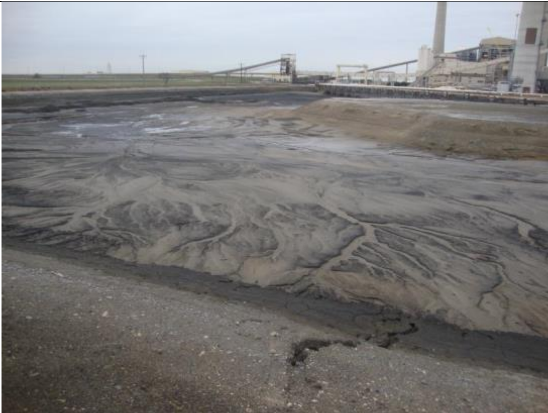
Photograph: 29 South Bottom Ash Pond – standing on eastern berm – facing southwest. Erosional features on eastern berm. Photo taken 12/20/16.
