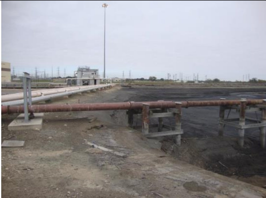
Photograph: 27 South Bottom Ash Pond – standing on southwestern corner – facing north. Photo taken 12/20/16.
