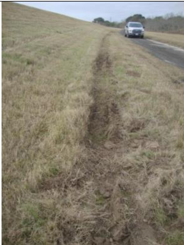
Photograph: 6 Fly Ash Landfill – standing on northern berm – facing west. Rutting at base of slope from vehicles. Photo taken 12/20/16.
