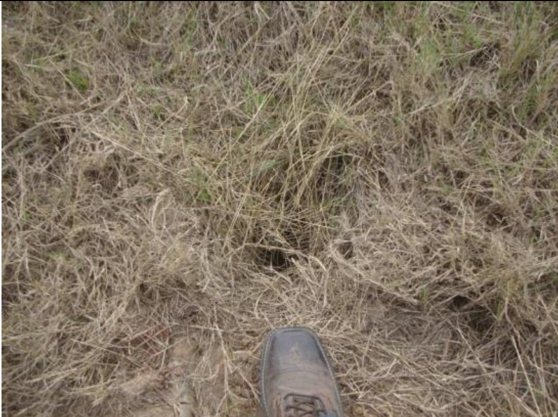
Photograph: 7 Fly Ash Landfill – standing on northern berm. Animal burrow in exterior slope. Photo taken 12/20/16.
