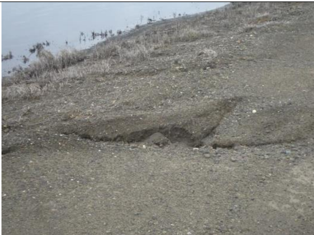
Photograph: 16 North Bottom Ash Pond – Erosion features on inside of eastern berm. Photo taken 12/20/16.
