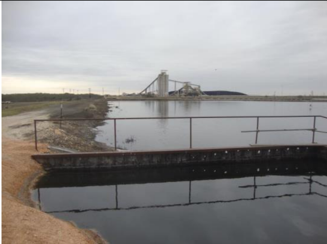
Photograph: 17 North Bottom Ash Pond – standing on northeast corner – facing south. Photo taken 12/20/16.
